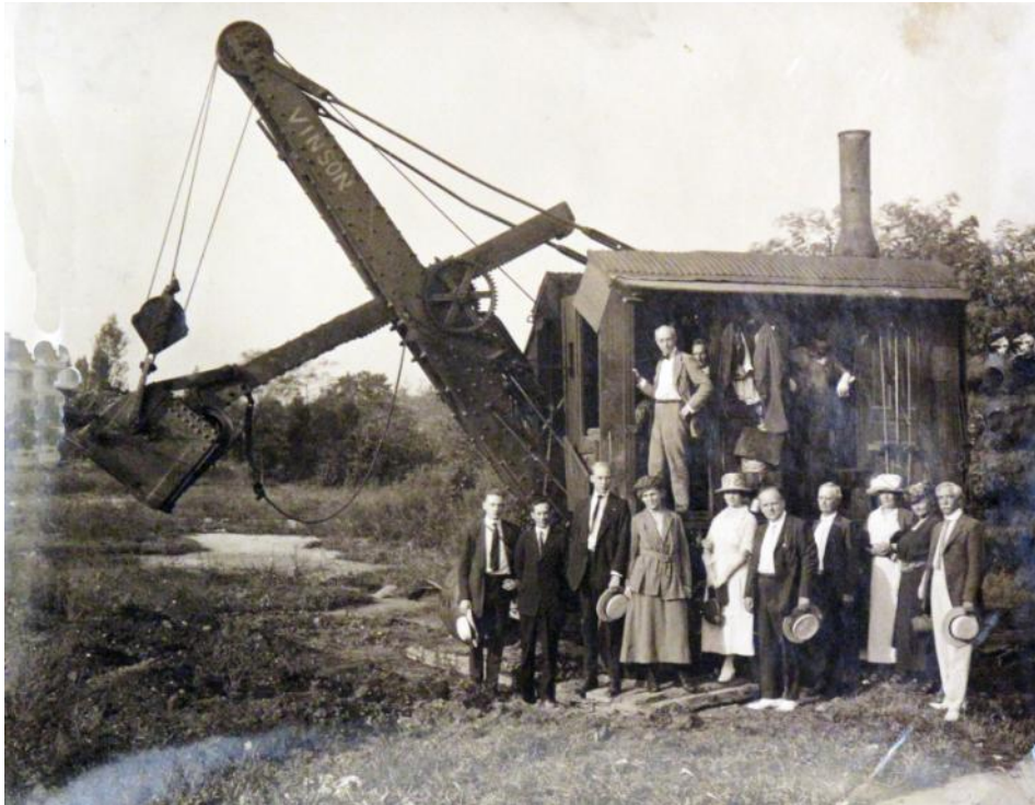
Breaking ground at 16th and Harvard Streets, 1921.
